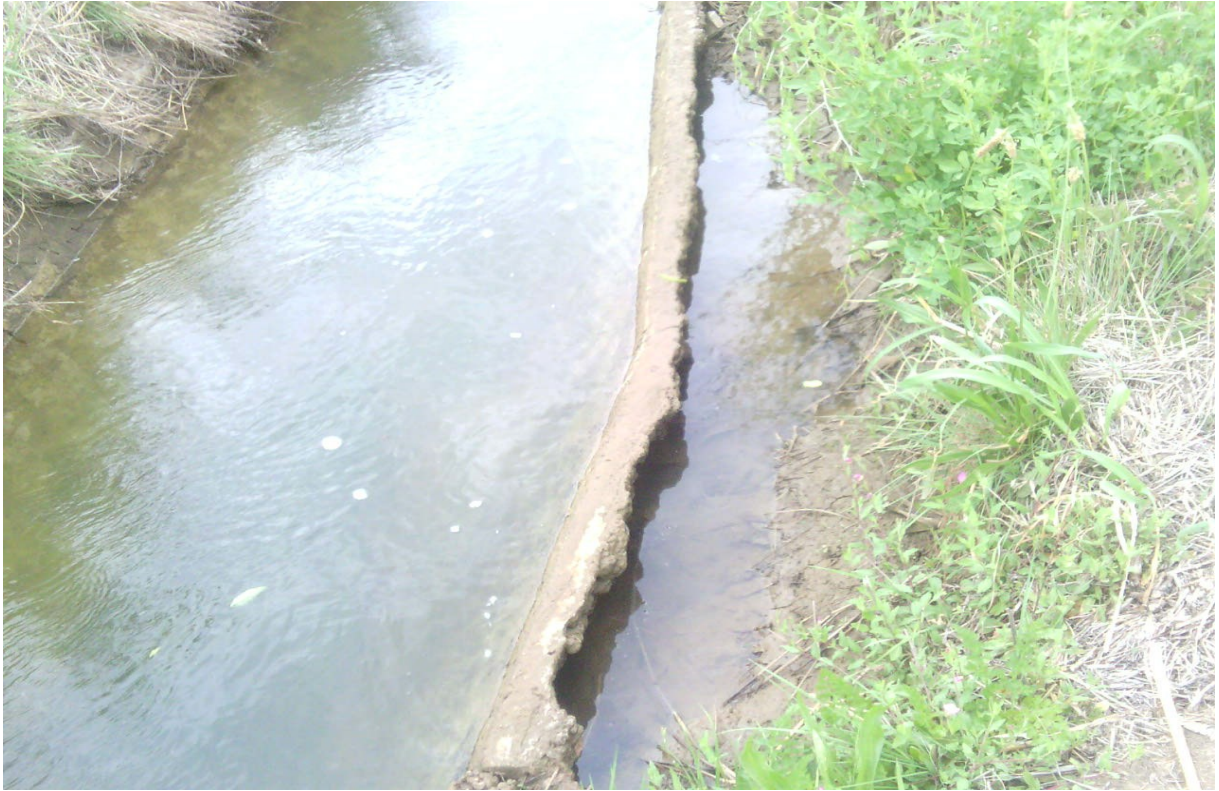
Photo 5:4: Canal leakage on the Lakeside canal
