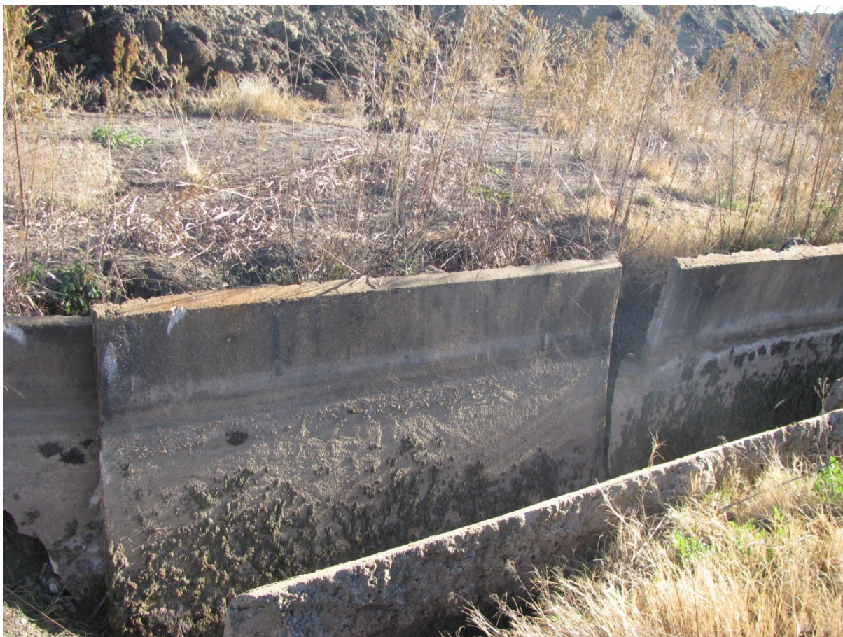
Photo 5:2: Photo of the Boskop Dam right bank canal illustrating the poor condition because of the expansive soils
