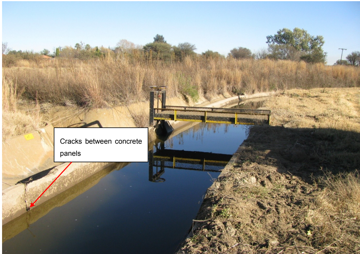
Photo 5:3: Cracks on canal concrete panels
